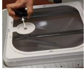
REMOVE THE HANDLE/CRANK
