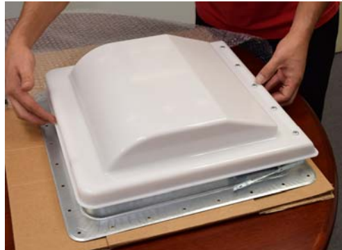
PUT LID ON AND PUSH BACK ON THE BLACK FOAM SPACERS
