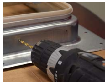
DRILL HOLES WHERE MARKS ARE
